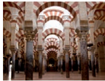
FIG. 1.18 Interior of the Mosque of Cordoba. In this Fig. the horseshoe arch use can be appreciated.
