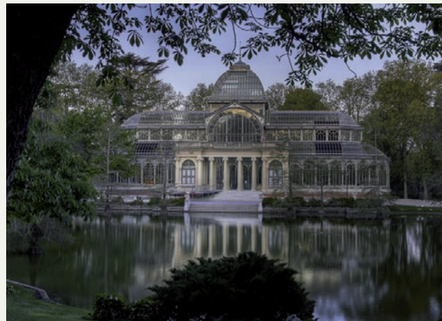
FIG. 3.17 The Crystal Palace venue for the Universal Exposition was built to display innovations of the Industrial Revolution. It contained the largest amount of glass ever used in a building, hence the name.
