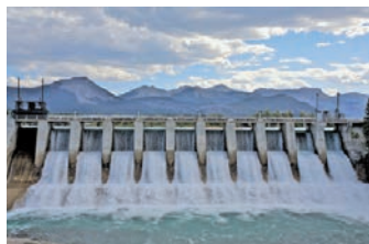
FIG. 4.53 A hydroelectric plant.
