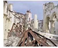
FIG. 5.13 Cathedral of Port-au-Prince, Haiti, after the earthquake.
