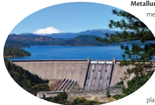
FIG. 4.5 Simon Bolivar hydroelectric central in Caroni River, Guyana.
