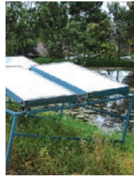
FIG. 1.10 Solar panels use sunrays to heat water for the house.
